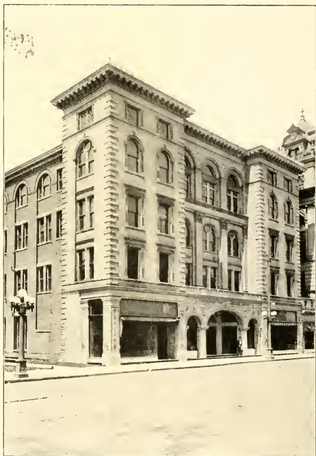
PIEDMONT FIRE INSURANCE COMPANY'S BUILDING
